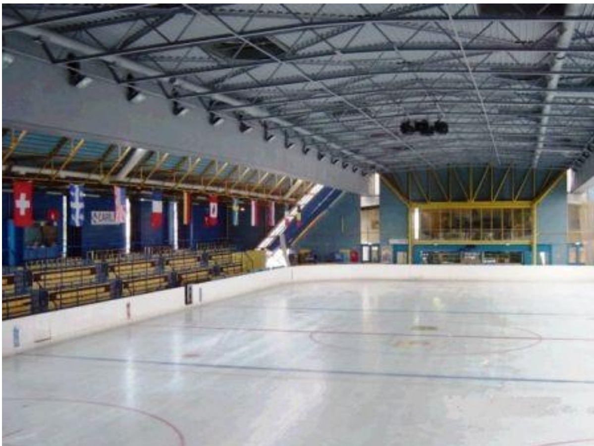
Paul Chemetov's buildings, built in 1979 which is Saint Ouen's (Paris' suburb) ice rink building. This ice rink is situated six meters above the ground and, thus, keeps traffic axis under. Building's structure is made with four posts carrying two 3,60 x 0,80m beams.
